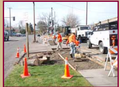
Crews work to replace sidewalk damaged by a street tree.
