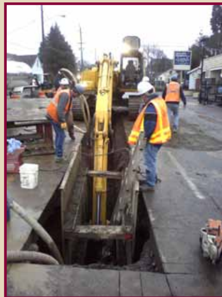
East Belmont Sewer Rehabilitation.
