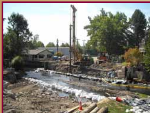
Capitol Street bridge before.
