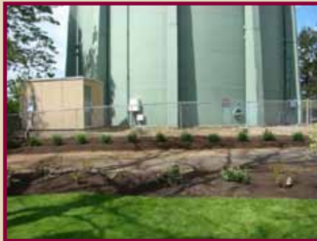
Mader Reservoir landscaping.
