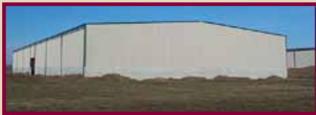
Biosolids winter storage facility.
