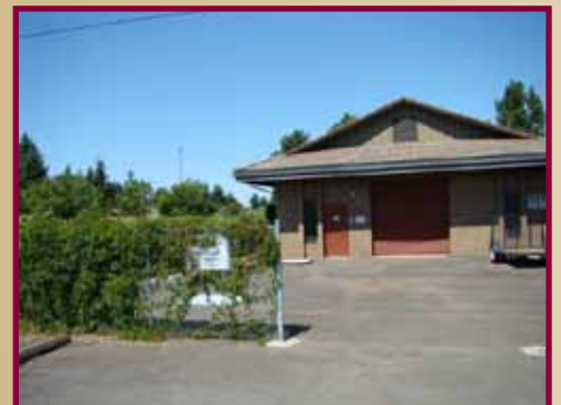
Boone Road Water Pump Station.
