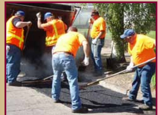
Maintenance paving crew at work.
