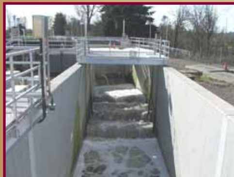
Willow Lake Water Pollution Control Facility effluent.
