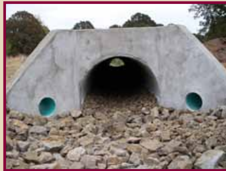
Gaia Street SE culvert in place.
