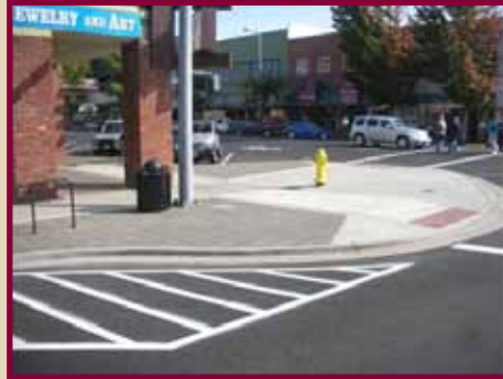
Commercial Street curb extensions.
