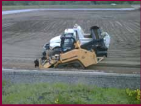
Slow sand cleaning.
