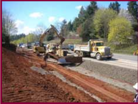
Kuebler Boulevard road widening.
