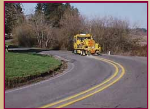
Crews paint traffic striping to improve safety.
