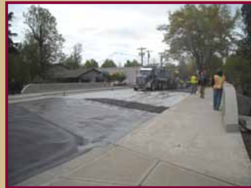
Capitol Street bridge after.
