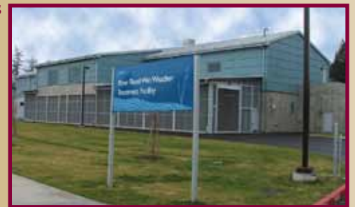
River Road Wet Weather Treatment Facility.
