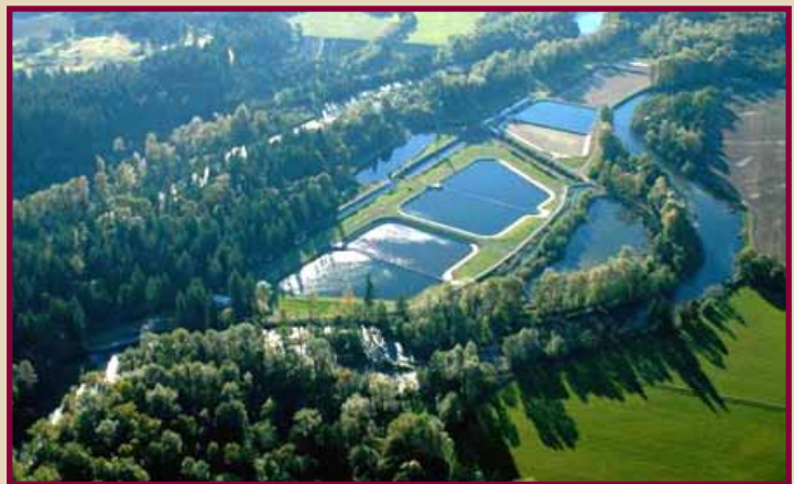
Geren Island Water Treatment slow sand filters.
