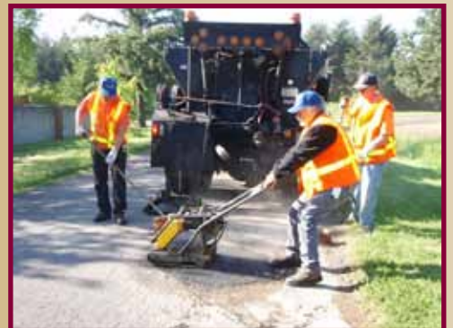
Crews finish patching a pothole.
