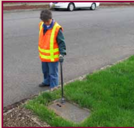
Water Meter Reader performing meter reading with wand device.
