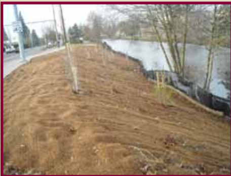
Cottage Bridge stream restoration.
