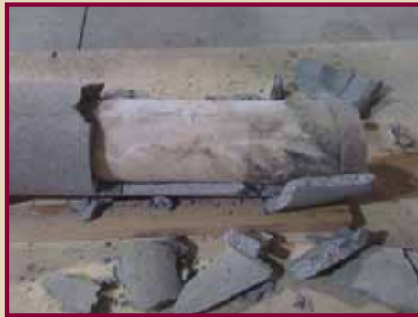
Example of a cured-in-place pipe liner; a no-dig technology that allows an existing pipe to be rehabilitated without digging up the street.
