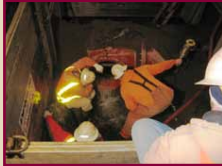
Distribution night work.
