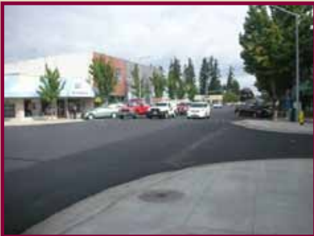
Commercial Street NE/SE—Marion Street NE to Ferry Street SE.
