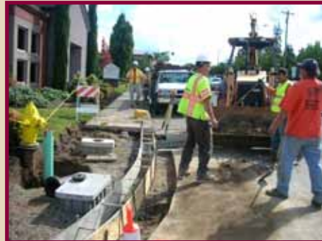
Commercial Street SE pavement RR.
