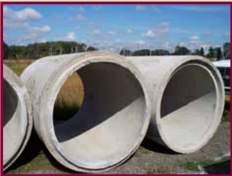
56-inch concrete pipe used at Gaia Street SE.
