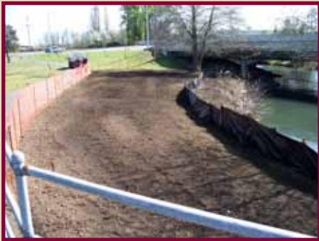
Preparing site for revegetation efforts.
