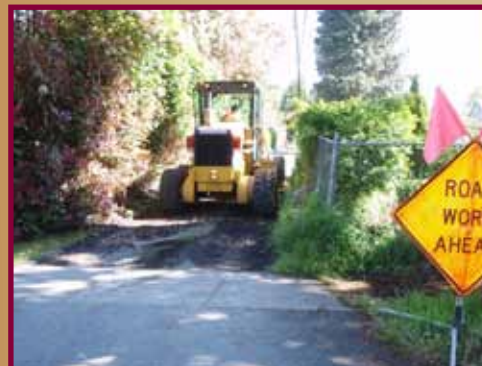
Grading a gravel alley.
