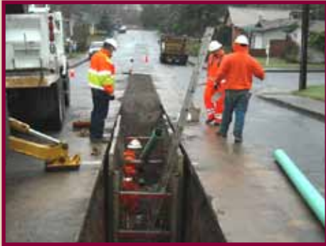
Dig and replace repair operation.
