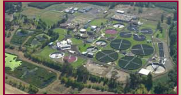
Aerial photo of Willow Lake Water Pollution Control Facility.
