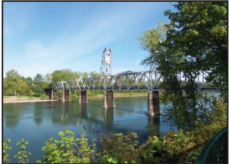
Union Street Railroad Bridge
