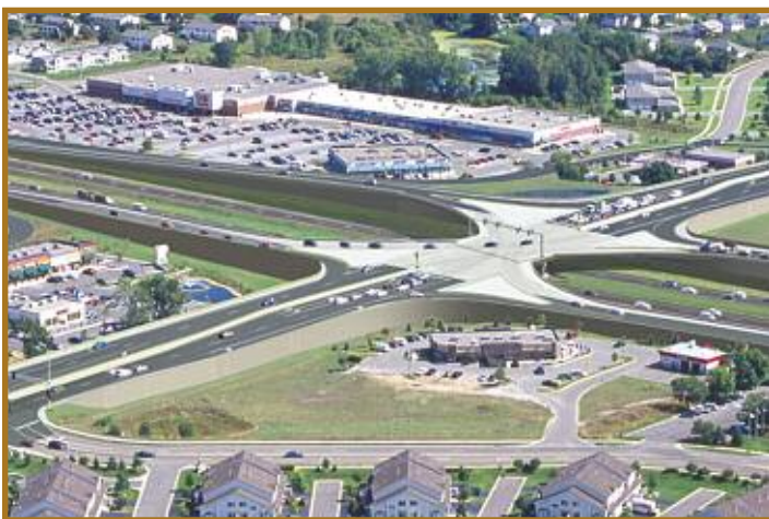
Through an extensive public involvement and outreach process the TH 65-CSAH 14 interchange improvement project met its goal of maximizing safety, capacity, and mobility, while minimizing disruption to the local businesses and residents.
