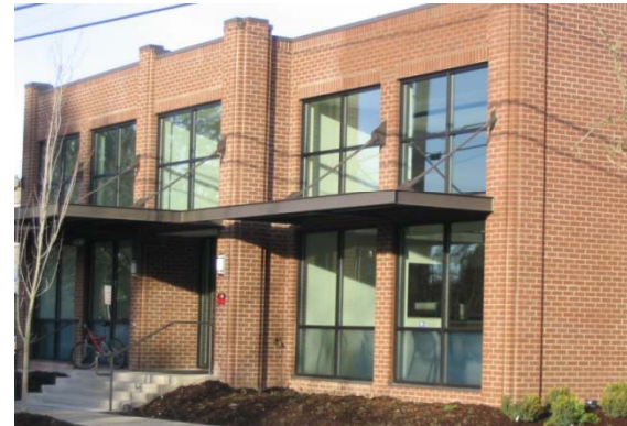
The old City Hall building on Edgewater is an example of a recent building rehabilitation project in the Area.
