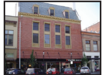
Salem Arts Building - Toolbox funded
