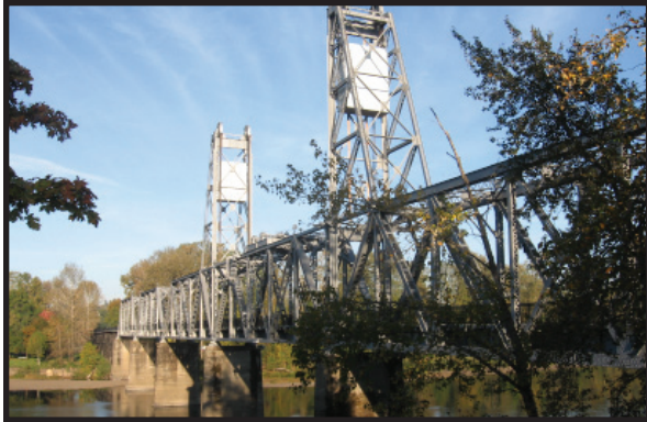
Union Street Railroad Bridge Conversion
