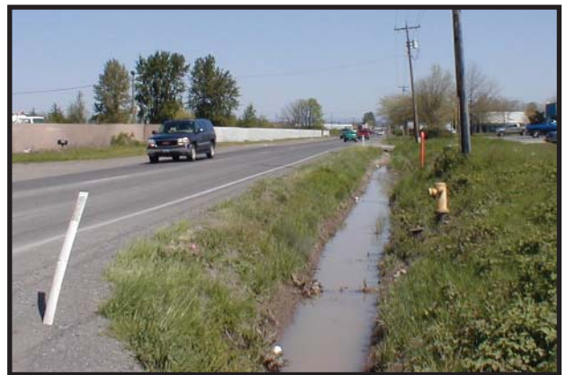
Existing Infrastructure - McGilchrist Street
