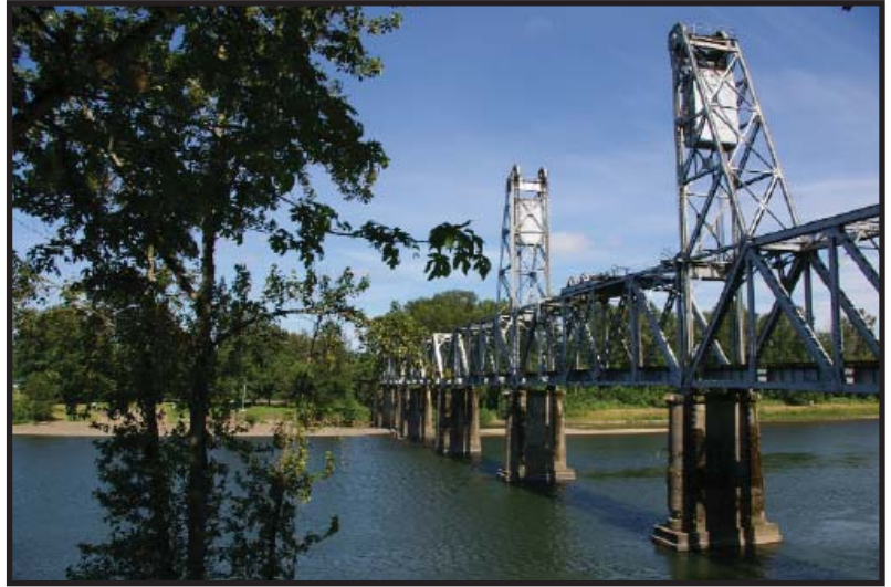
Union Street Railroad Bridge Courtesy: Oregon State Historic Preservation Office
