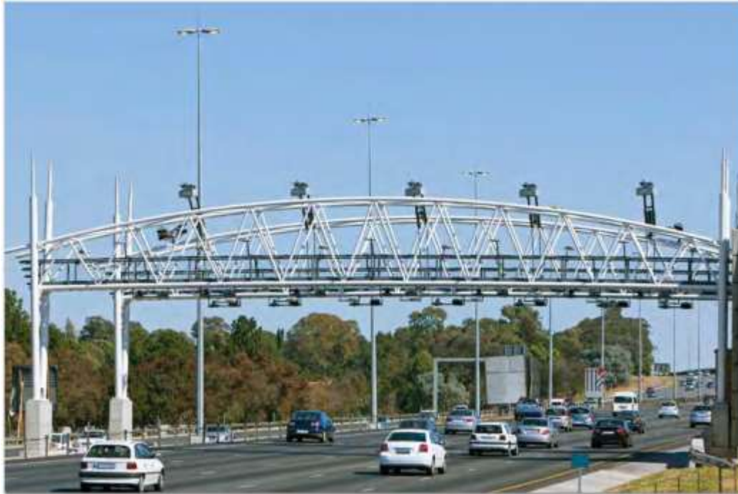
Figure 1: A typical tolling gantry installation 10
