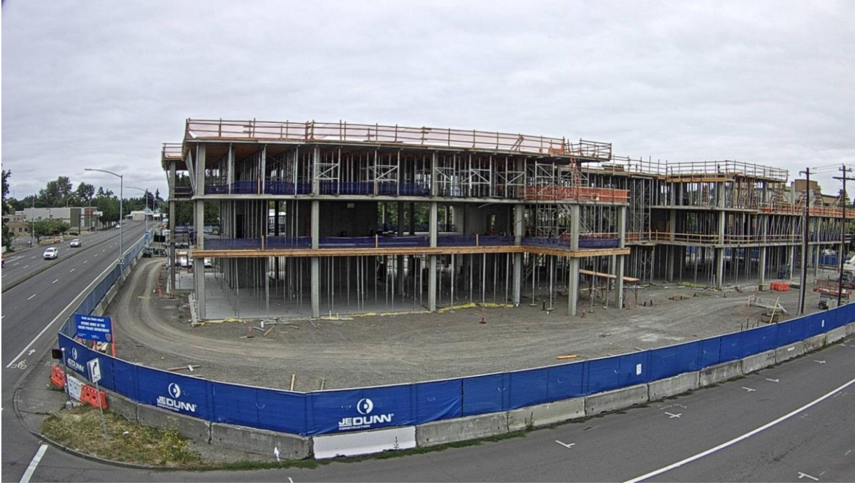
View From Police Station Project Cam – July 5, 2019
