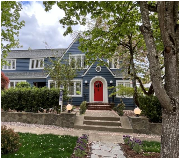
460 Bush St SE after restoration
