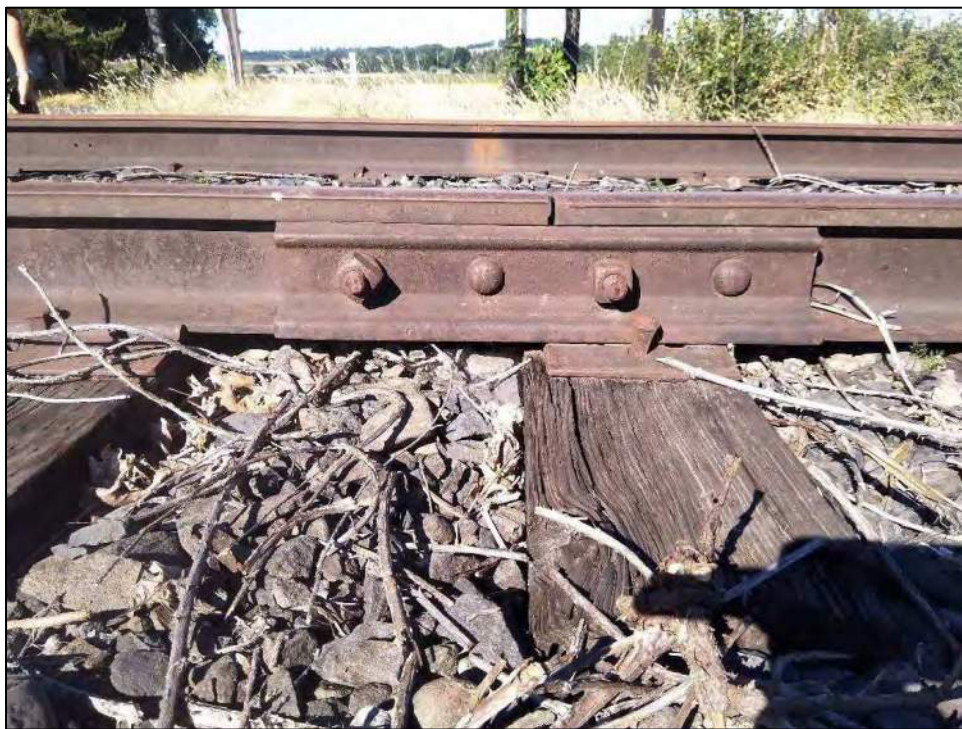
Figure 64. Profile of railroad tracks.
