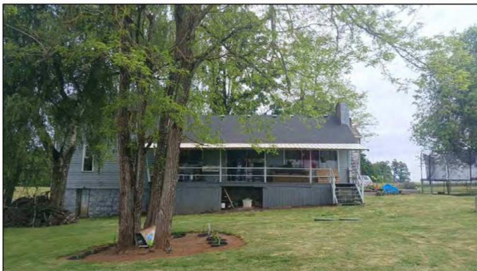
Figure 54. Overview of TS01, facing south from shovel test IP1016.
