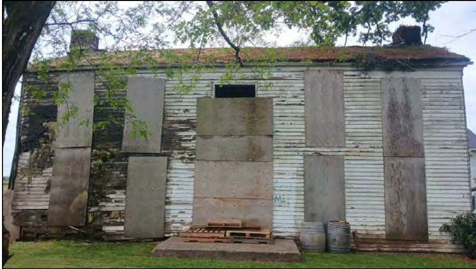
Figure 51. View of the Daniel Waldo House, facing west from entrance façade.
