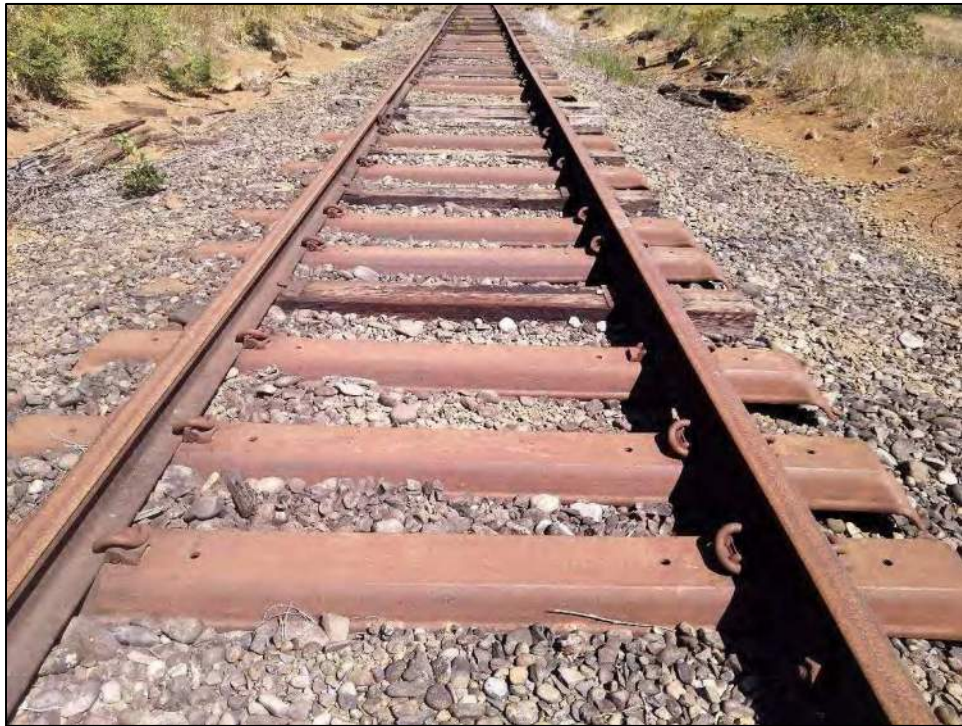
Figure 65. Overview of metal and wooden ties.
