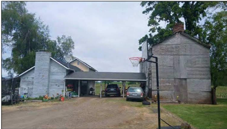
Figure 53. Overview of TS01 with the Daniel Waldo House and adjoining structure.
