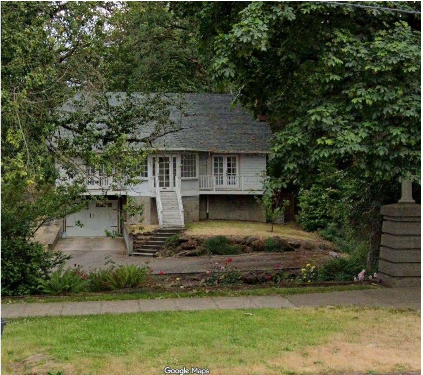
View of property from Church Street. Lot setback is approximately 70 feet.
